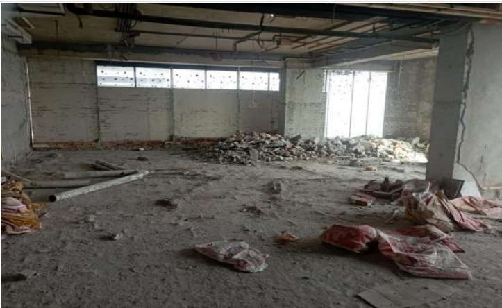
L-14-Kitchen Area on 24-10-23
