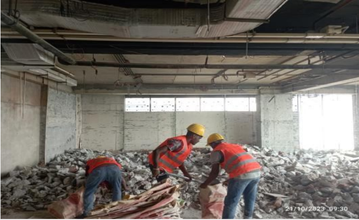
L-14-Kitchen Floor Debris Removing on 23-10-23
