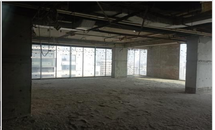
L-14-Old Kitchen Area on 25-10-23
