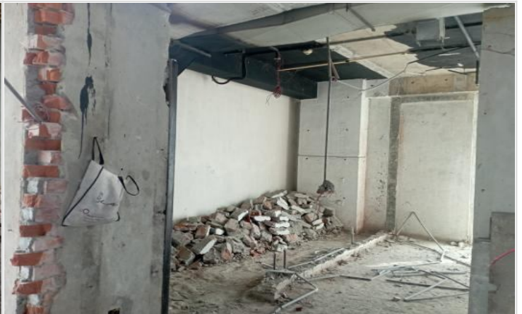
L-14-Kitchen Area on 24-10-23
