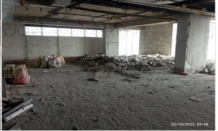
L-14-Kitchen Area on 23-10-23
