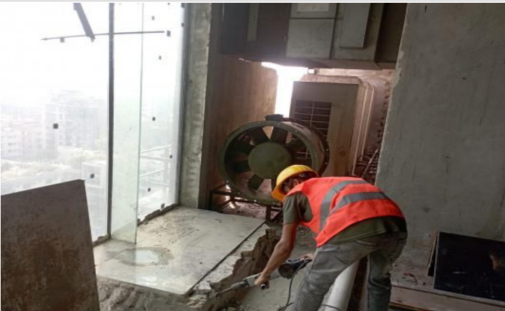
L-14-Old Kitchen Floor Dismantling on 25-10-23
